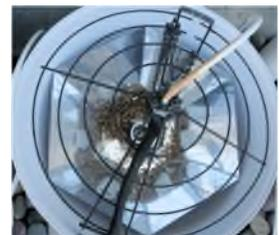
lighting fixtures. *Pictured Right: is a Indirect Halide that was removed however there was about 1/2" of bugs and dirt built up after 2 years since cleaned*
